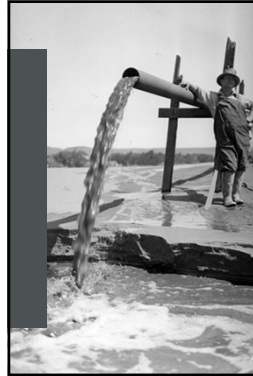
Photo: George Hager stands near a pipe that drains the sand, water, and tailings mixture from the Golden Cycle Mill in El Paso County. Source: The Gazette
