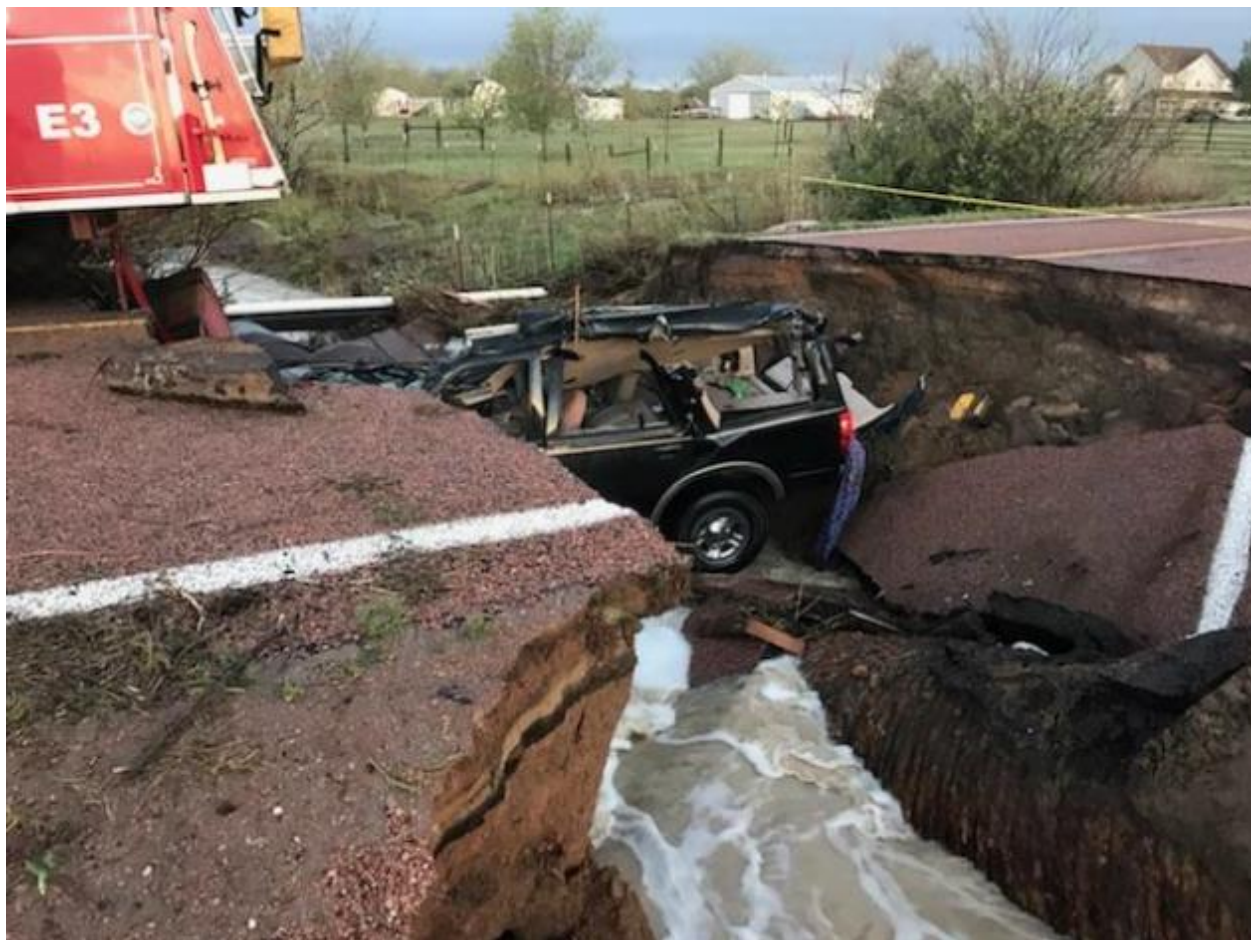
Figure 4-47: Old Pueblo Road After a Sinkhole Trapped Two Cars and a Firetruck on July 24, 2018
